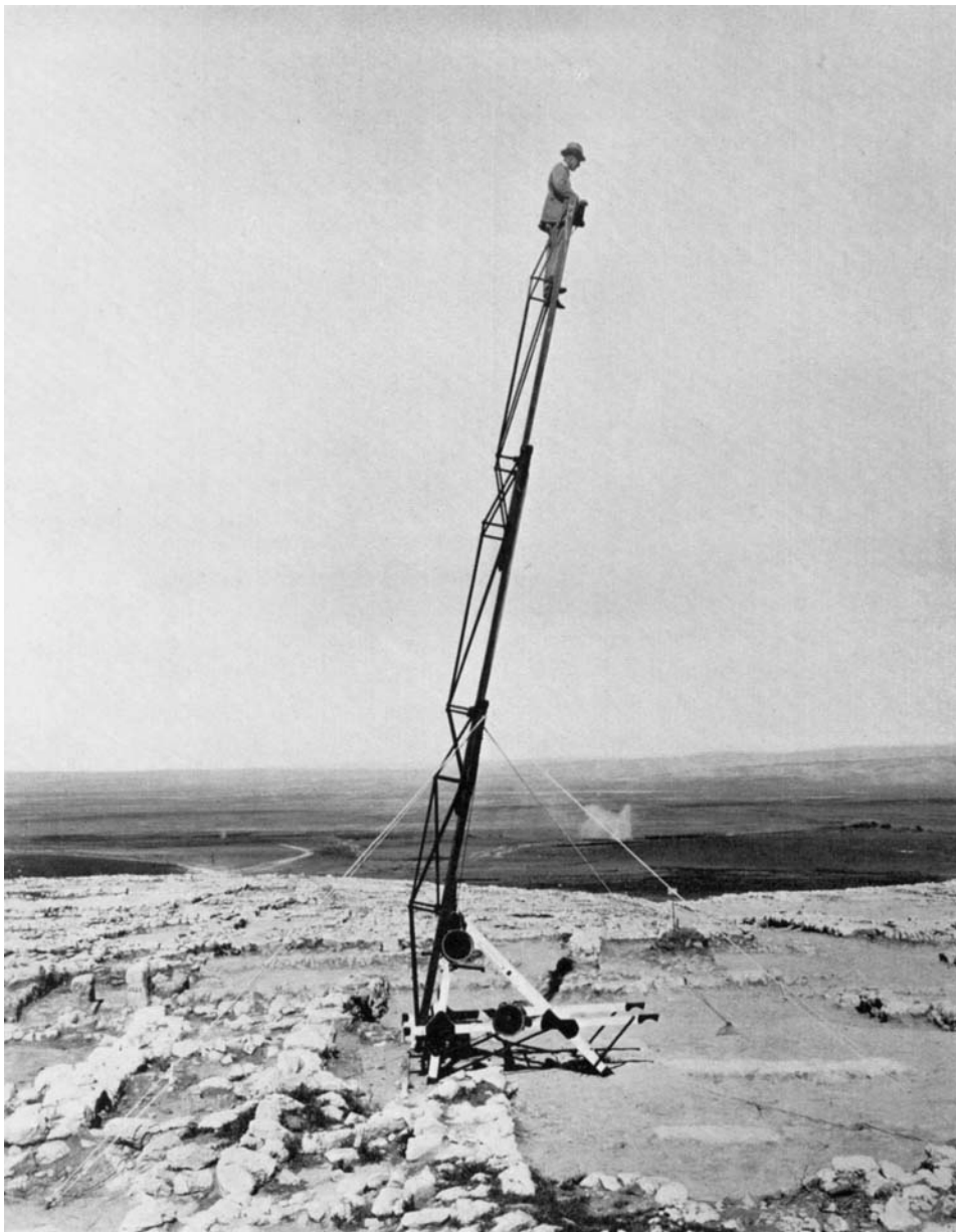
EXTENSIBLE LADDER USED AT MEGIDDO FOR OBSERVATION AND PHOTOGRAPHY
