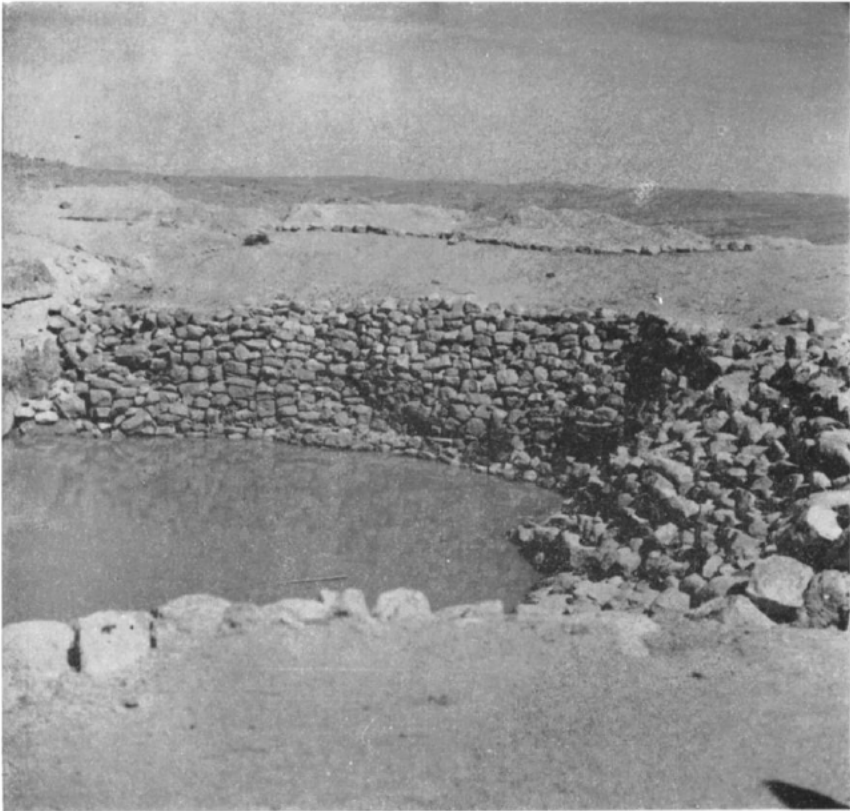
Fig. 7. Judean kingdom cistern in the Negev, still watertight, with water from rains of February-March 1959. Photo: Nelson Glueck.
