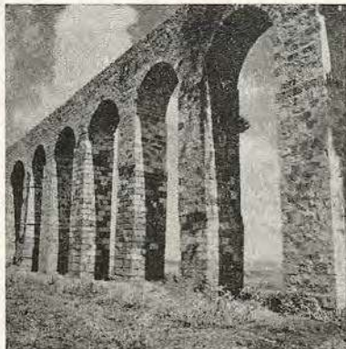
2. Another view of the aqueduct.
