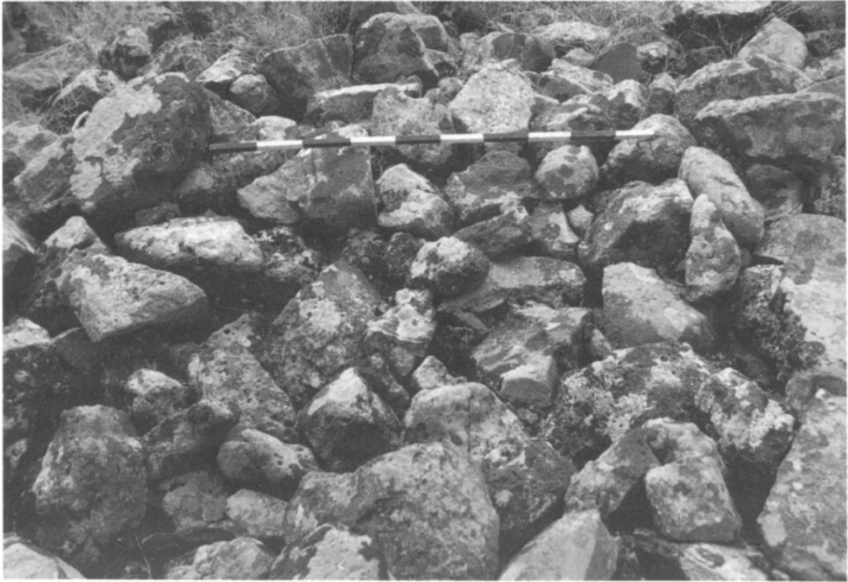
Fig. 3. Debris of outer EB wall at Leviah. Large lichen colonies cover stones.
