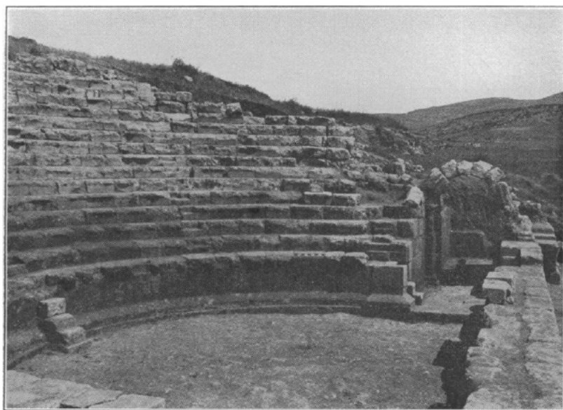
Fig. 7. The Little Theater, north of Jerash. A portion of the seats, with the north public entrance. On the right the front wall of the stage.
