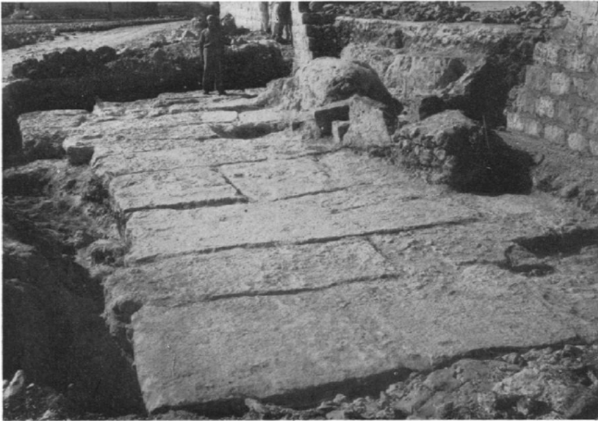
Fig. 1. The footings of the Third Wall as found outside the property of the Schools and below the new street. At the left can be seen the continuation of the Third Wall eastward.
