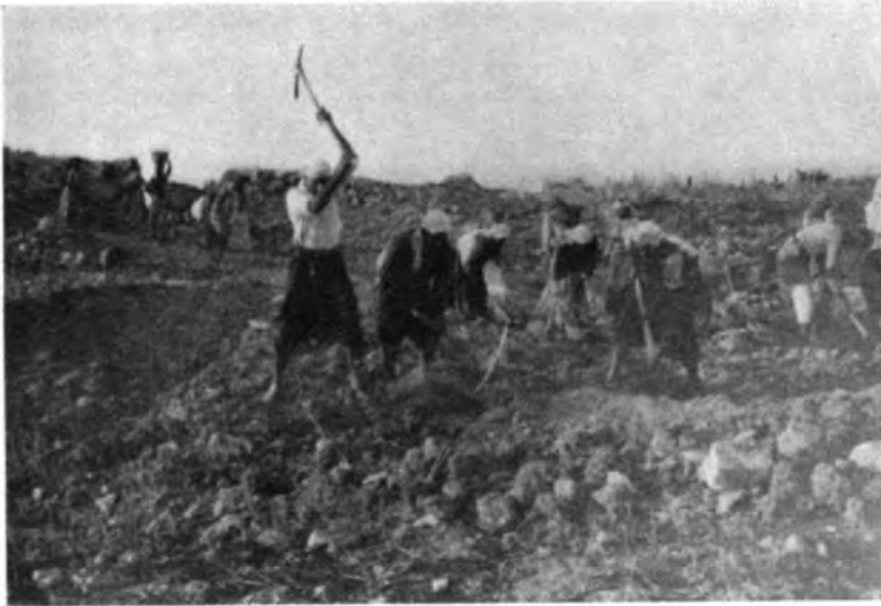
FIG. 12.—Pickmen breaking up the surface layer of earth
