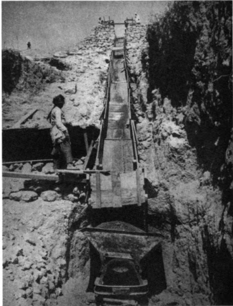
FIG. 37.—The lower end of the wooden chute, with a loaded car ready to be wheeled out upon the dump.
