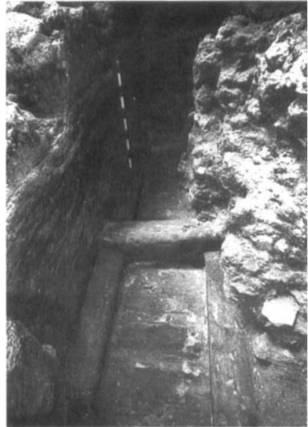
Figure 10. An inner wooden chamber with frames and mortised floor, part of the rectangular barge that was built as a forming device for the artificial island at the base of the lighthouse in area K-2 (no. 32).
