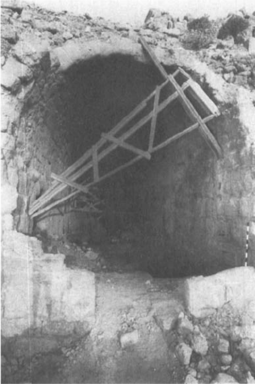
Figure 16. The great vault at the south-west side of the Herodian podium, looking east; notice the different type of structure of its side walls (M. Little).
