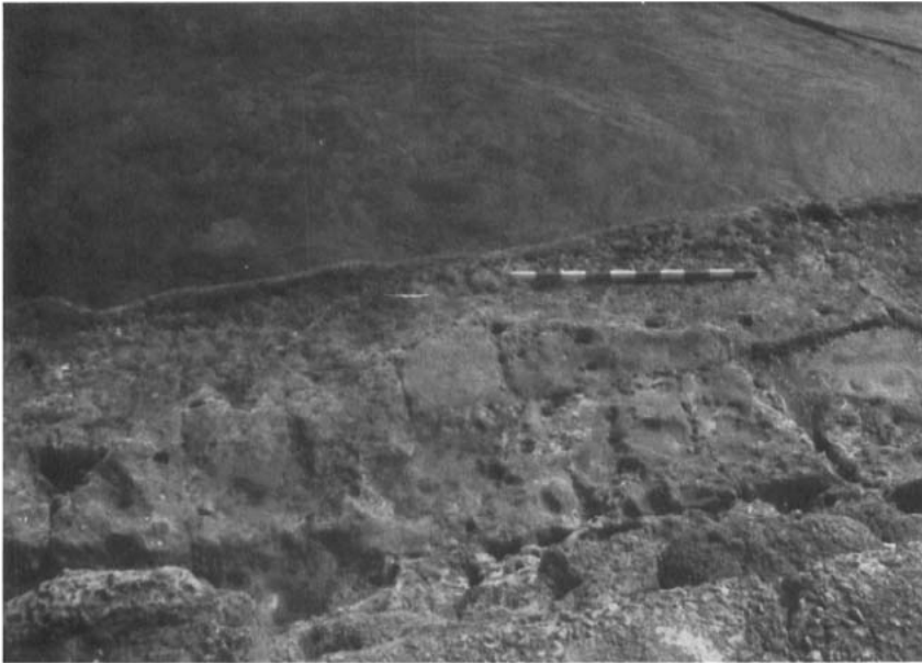
Figure 9. The top of the Herodian (?) inner quay at area Q and the Crusader and modern structures on it.
