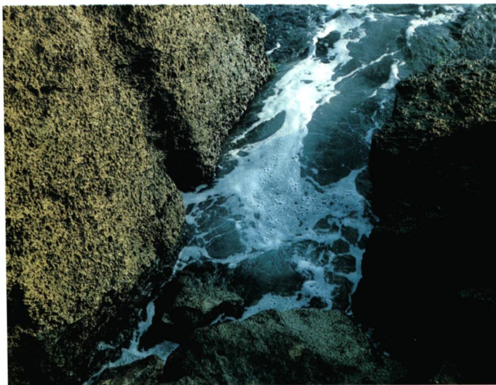
Sluice gate used to help control silting within the harbor on the southern Herodian breakwater.
