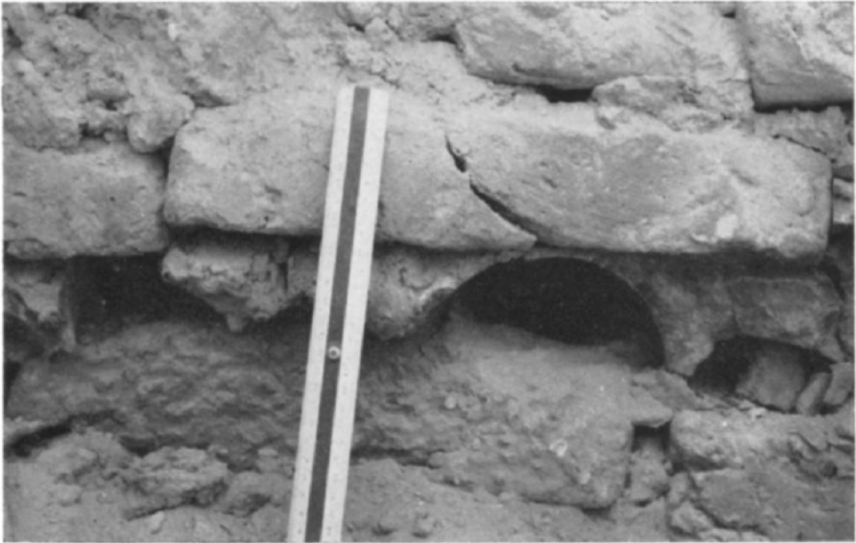
Fig. 3. Close view of apertures in the mudbrick walls; conceivably they served for ventilation, but their basic purpose was for bonding.
