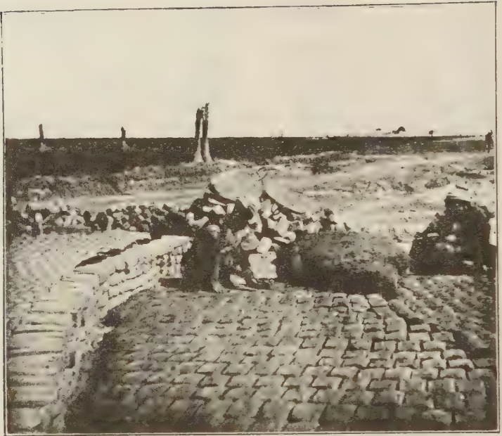
FIG. 11.—Modern Egyptians making bricks. Note the mat beyond the man for carrying the mud, the mould of mud, the water-pot for wetting the mould, the rows of bricks drying on the ground, and the dry bricks stacked on the right.
