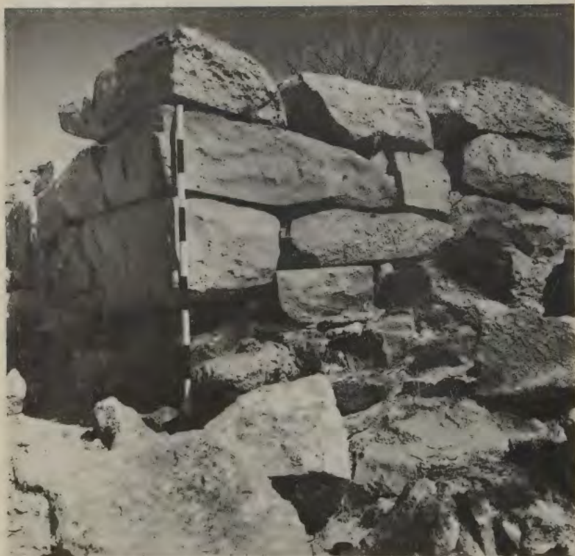
FIG. 24. Cornerstones of a fortress of the Judaeen kingdom, showing typical header and stretcher bonding (see page 106).
