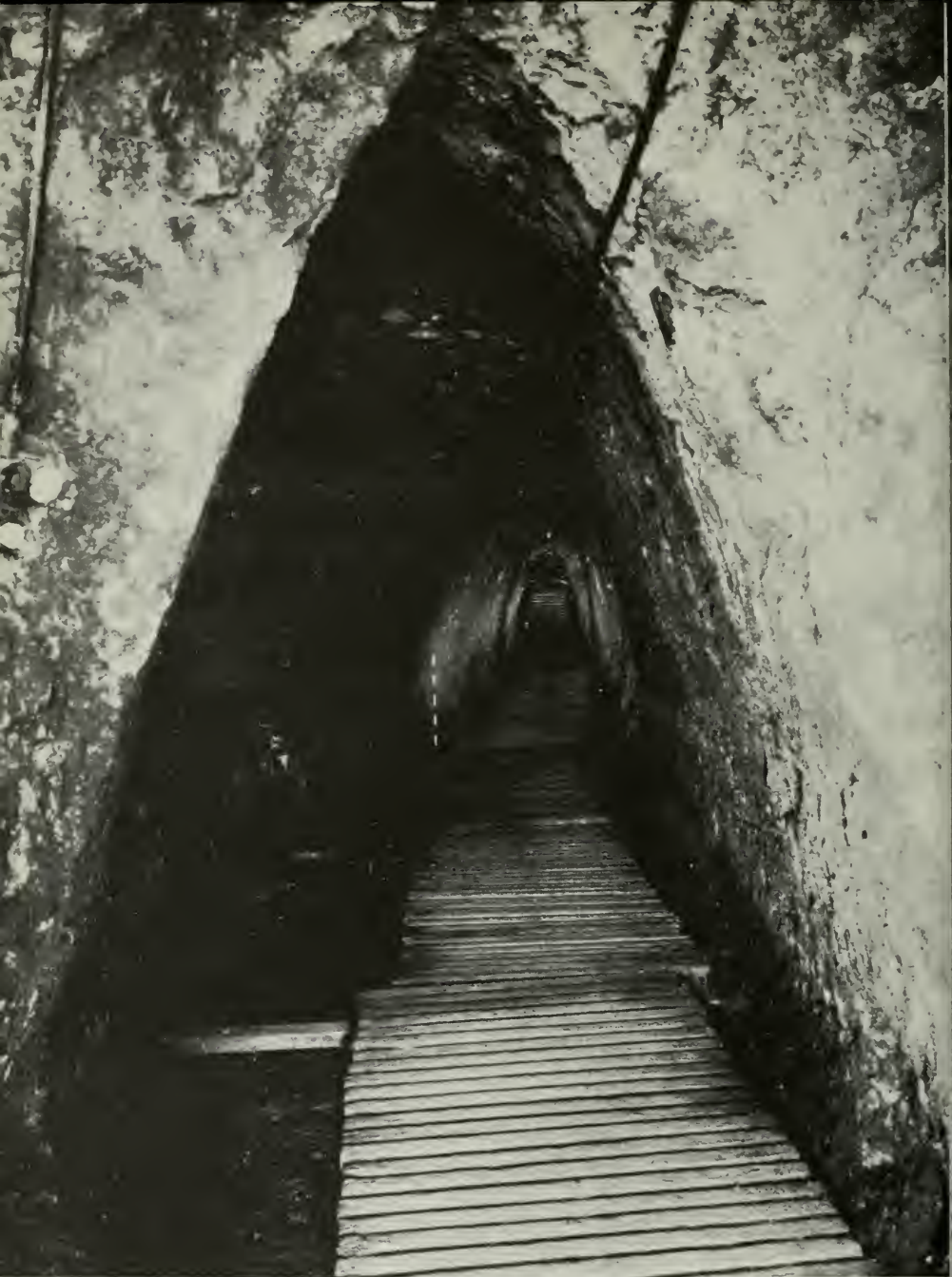
48 The tunnel from the shaft to the spring at Megiddo (p. 234)
