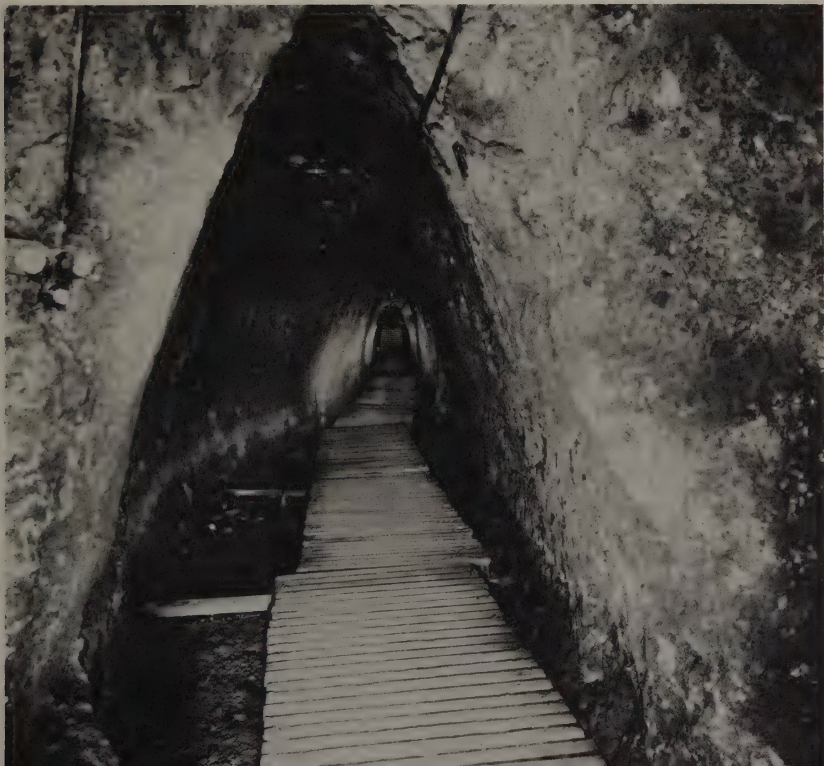
Pl. 70. Tunnel to spring at base of water shaft.
