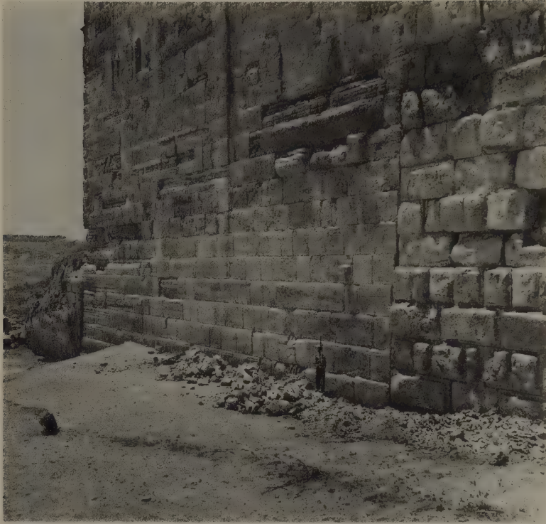
Pl. 17. South-east corner of Herod's Temple platform, with straight joint between Herodian and earlier masonry.
