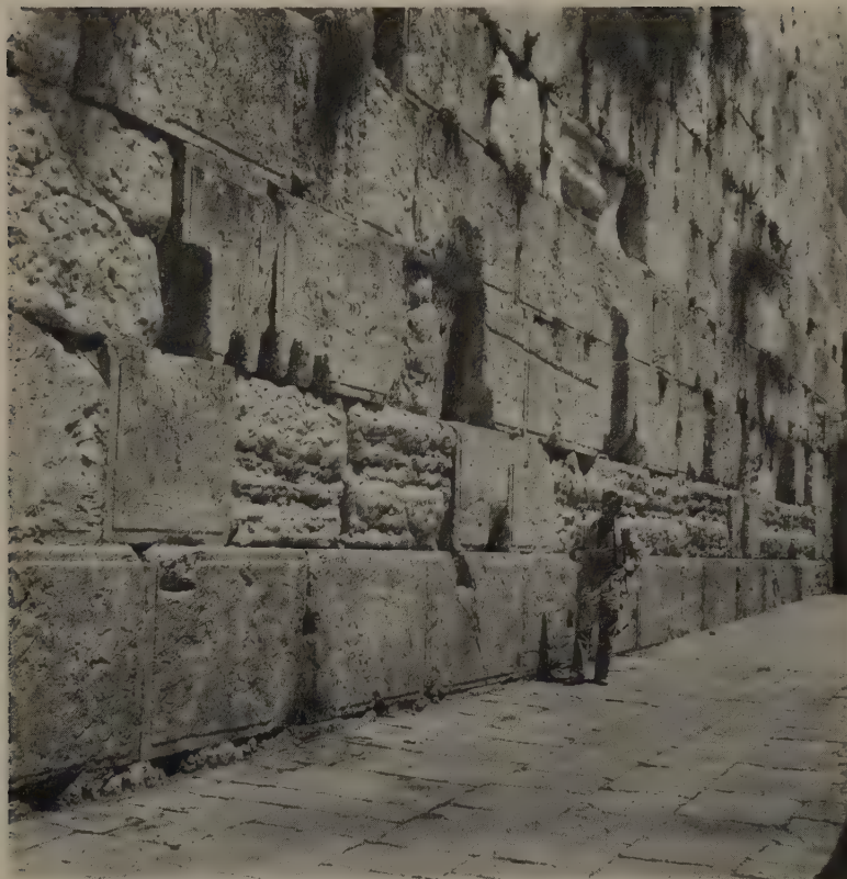
Pl. 19. Herodian masonry at the Wailing Wall at the west side of the Temple platform.
