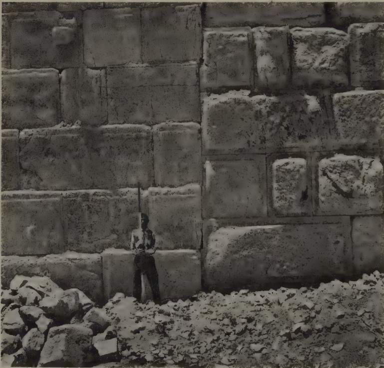
Pl. 18. Detail of straight joint between Herodian and earlier masonry.
