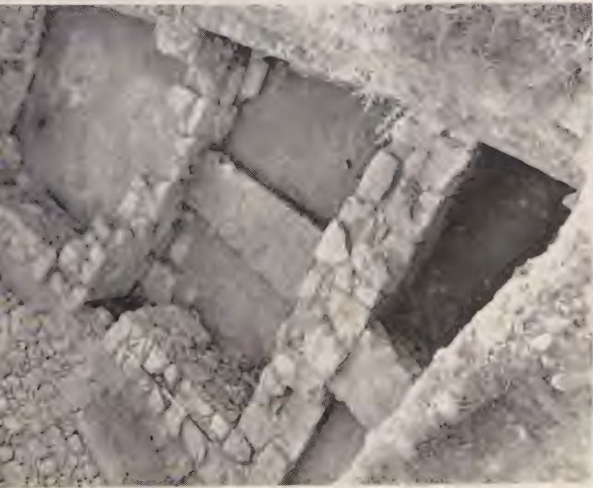
111 Part of a Byzantine house at Site A (p. 271)
