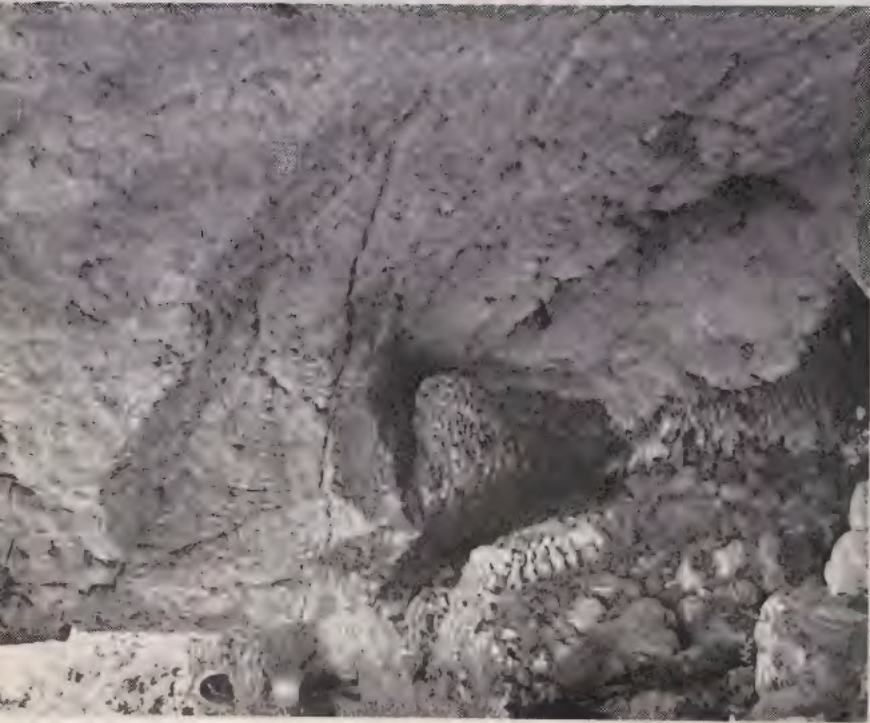
69 Original rock-cut channel carrying the overflow from the Pool of Siloam, of which the left-hand, western, wall has been removed by later quarrying (p. 159)
