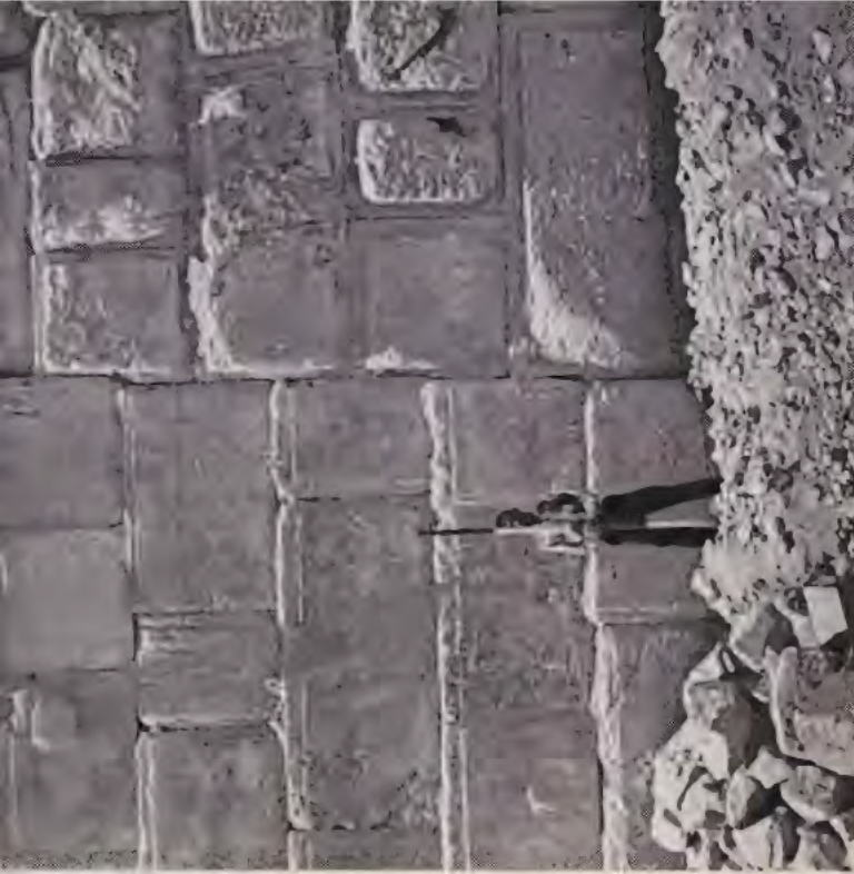
36 Detail of the straight joint between the Herodian masonry on left and the earlier masonry on right (pp. 111-12)
