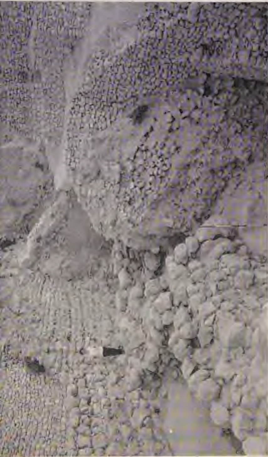
43 Left foreground, original wall N of Jebusite-D III c period, with angular return to west. Original wall is seen disappearing beneath later wall, N of 144-7th century (pp. 144-7)
