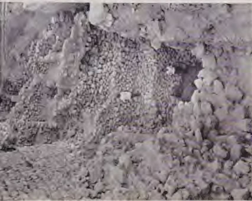
25 Stone-filled terraces constructed by Ishtar, 11th century B.C. Ishtar's right, retaining wall, against which a compartmented fill of stones shown in photograph, served to build up a terrace (p. 95)
