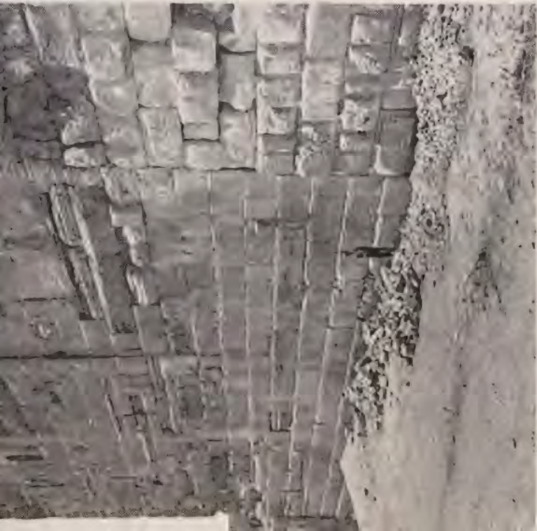
35 On left, Herodian masonry of temple platform. Between this and more heavily-bossed stones on right, a straight joint. The heavily bossed stones are in Persian style
