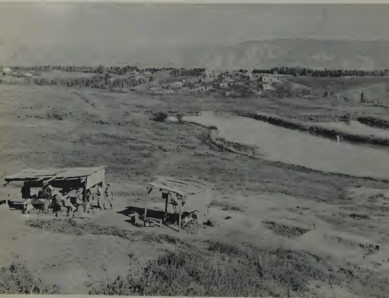
General View of Site A
